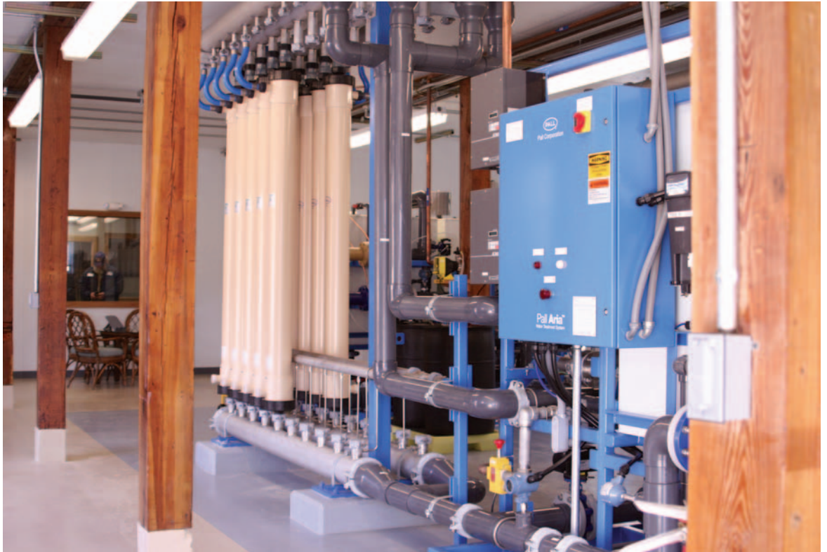
The Pall Aria system's microfiltration modules deliver consistent performance with minimal maintenance.
