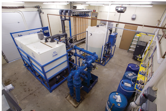
The Village of Groton, NY selected a Pall Aria AP system for drinking water treatment in their community.
