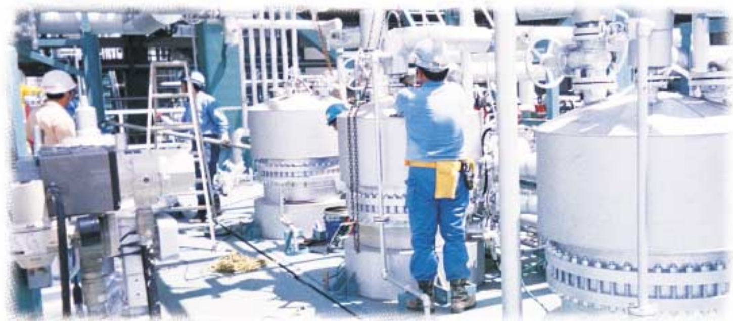
Refineries receive high return on investment after installing Pall backwash filters to protect catalyst beds and to remove catalyst fines from FCC slurry oil.
