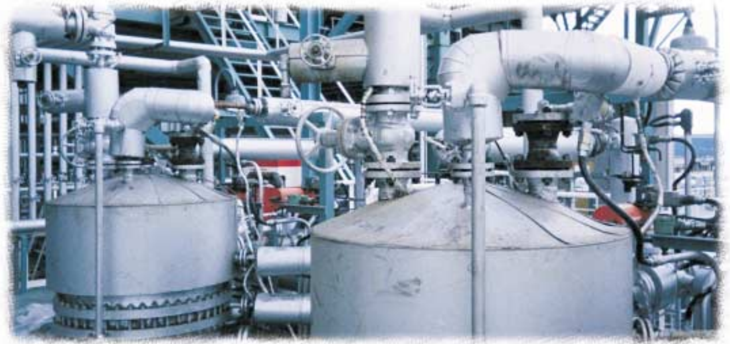
Pall blowback filters are used to remove catalyst fines from vent gas.
